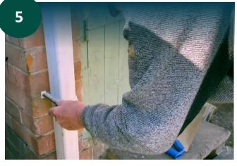
Make sure you secure a bracket to your wall and downpipe. You will need a drill and a screwdriver for this step.
