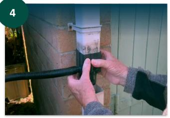
Attach the rainwater diverter fitting to the cut section of the downpipe. Make sure you follow the diverter kit instructions.
