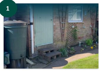
First, you'll need to find a flat surface near a gutter downpipe. Use a spirit level to check as this is where your water butt will sit.
