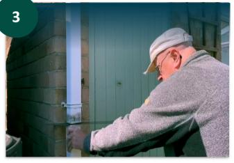
Mark the height of the water butt on the downpipe. Then measure 3 cm above this point, this is where you will want to cut with a saw.
