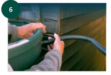
Attach the flexible hose from the diverter fitting to the water butt. You can cut this down to size if it is too long using a saw. 03
